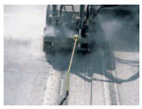
Optional guide rod available for 14", 16", 18" and 24" Bobcat planers; helps the operator maintain a straight cut.
