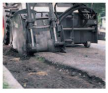
The **oscillation** of the planer provides optimum surface tracking and isolating the planer from loader movements caused by uneven terrain. Adjustable depth skis allow tapering of cut, such as when matching two uneven pavement surfaces or removing a curb ridge.
